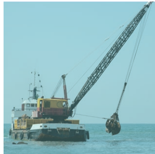
Dredging and Sediment Removal
